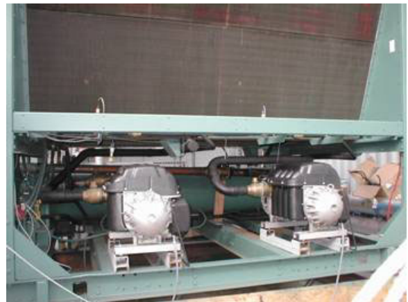
Figure 15. After – 120 Ton Retrofitted Chiller
