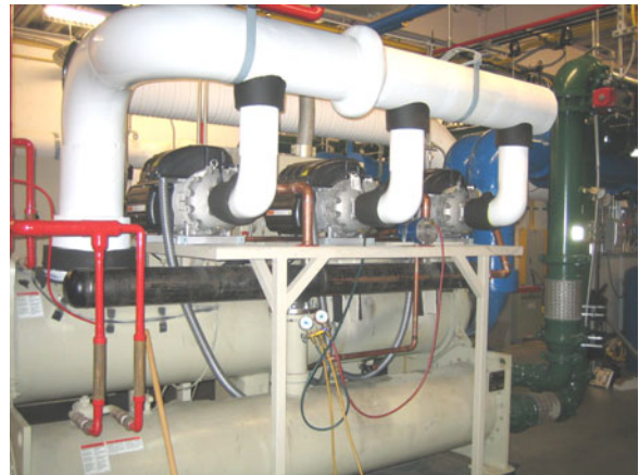
Figure 13. After – 250 Ton Retrofitted Chiller
