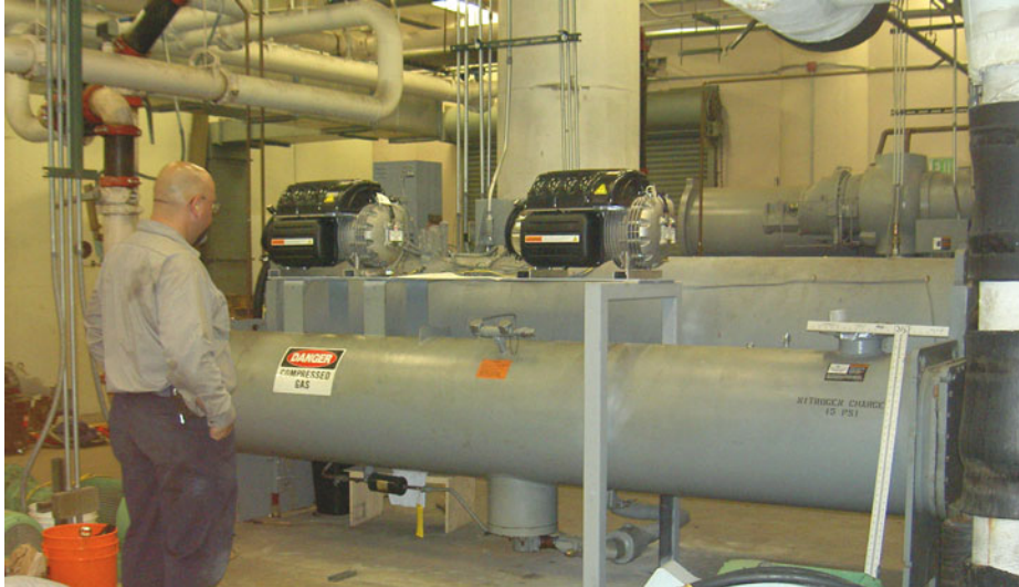
Figure 4. Post-Retrofit of Oil-less Compressors
