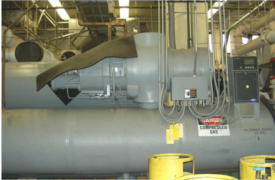
Figure 4. Post-Retrofit of Oil-less Compressors
