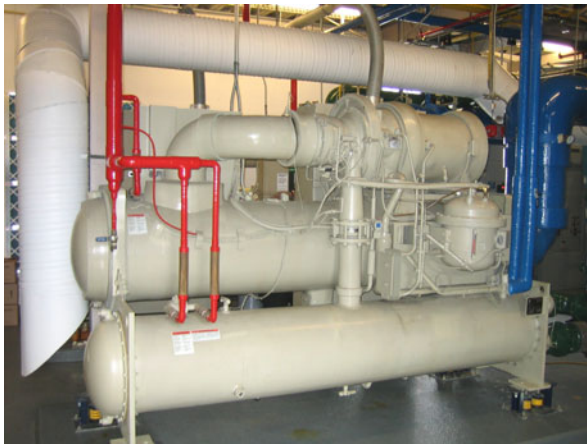
Figure 12. Before – 250 Ton Centrifugal Chiller
