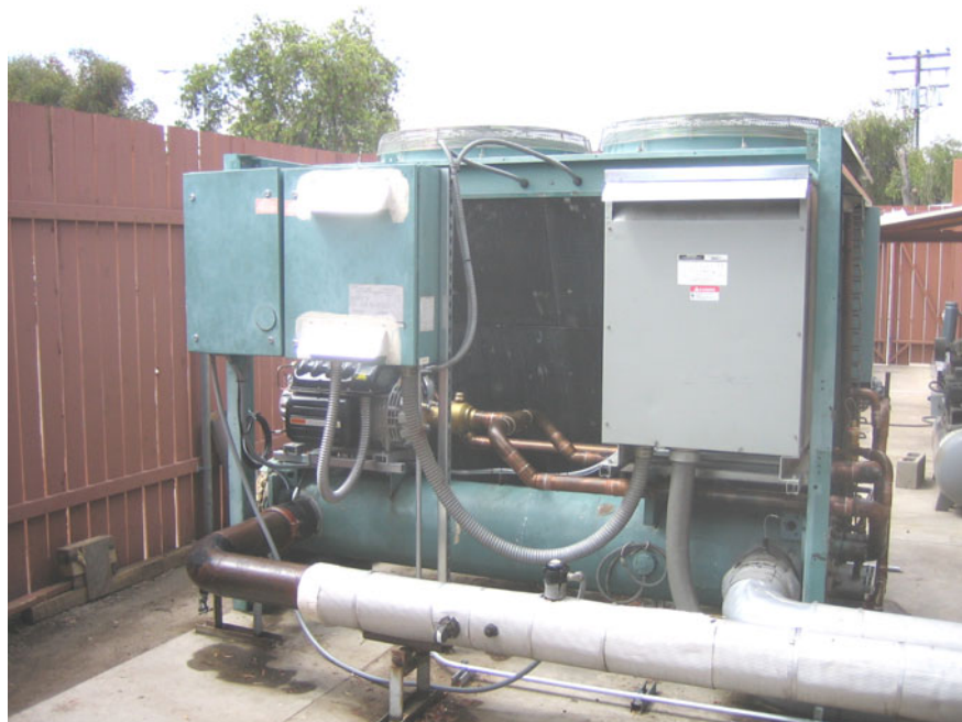
Figure 9. Air Cooled Reciprocating Chiller Post Retrofit
